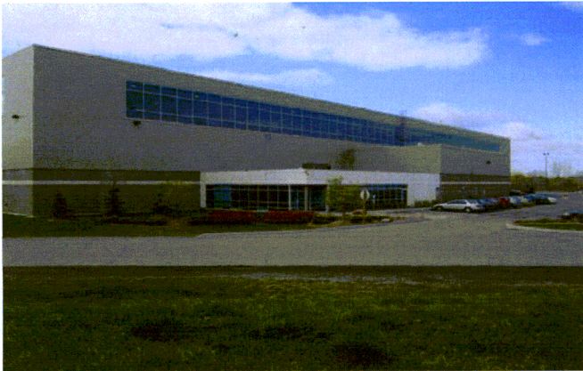
Material Recovery Facility, Whitby
